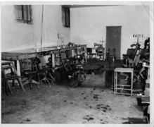
04.Warehouse after rain
